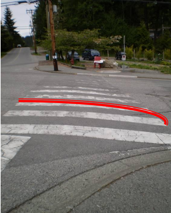
Crosswalk on speed bump, no curb cuts, difficult for walkers, wheelchairs and people with poor balance
