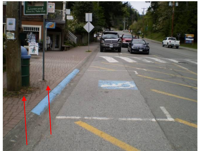
Handicap parking, can't open passenger door, no curb cut for wheelchair
